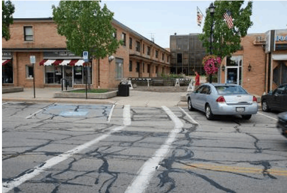
North Curb Ramp
