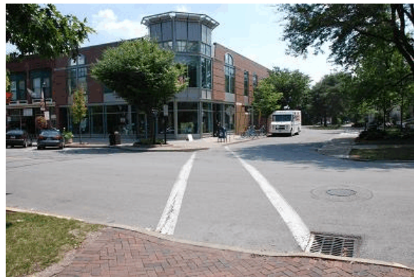
South Curb Ramps
