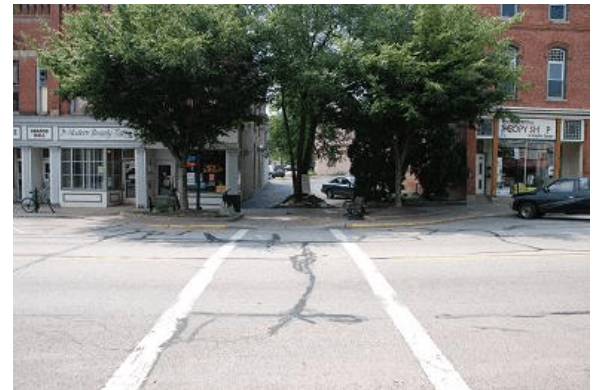
West Curb Ramp
