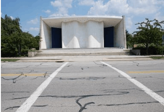
East Curb Ramp
