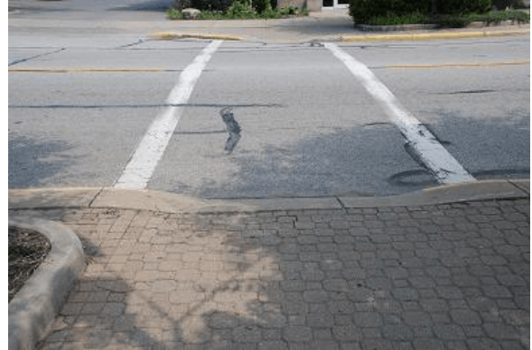
West Curb Ramp
