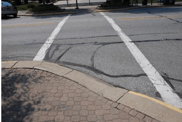
East Curb Ramp
