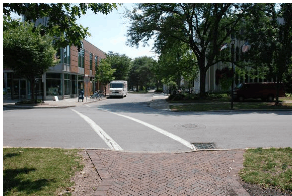
North Curb Ramp
