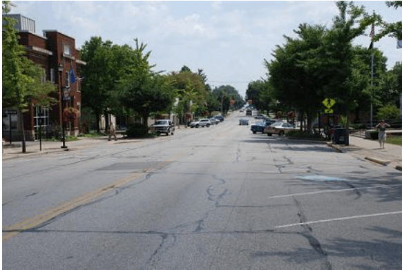
Old City Hall Looking South
