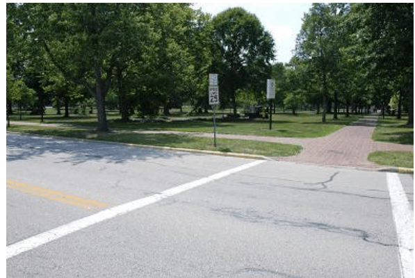
West Curb Ramp
