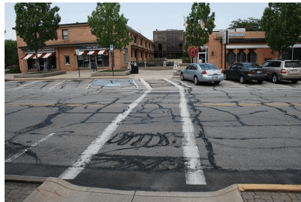
East College Crosswalk
