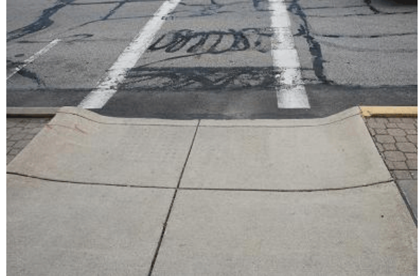
South Curb Ramp
