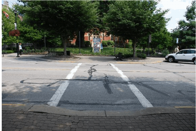
South Main Crosswalk Looking East
