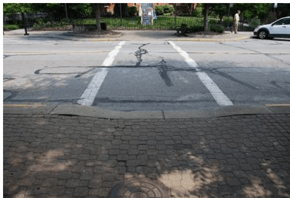
East Curb Ramp
