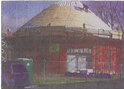
Repairs to the gasholder building began with the roof this fall.
