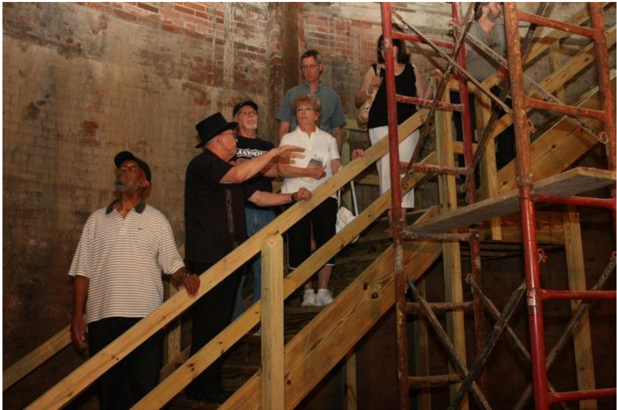
With phase one of the restoration process almost complete, the community was provided with a sneak peek of the Gasholder Building during an open house over commencement weekend.
