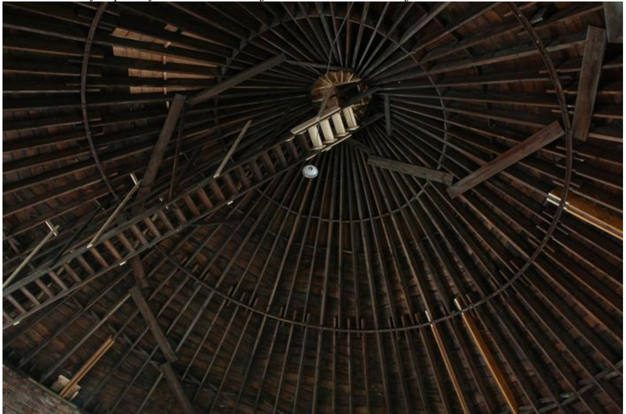
The Gasholder Building's roof seen from the interior of the building.
