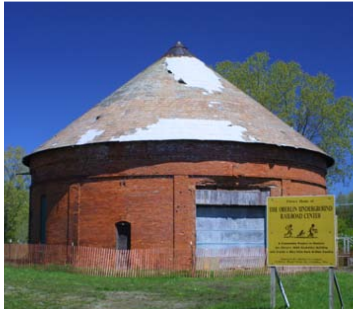
GASHOLDER BUILDING, FUTURE HOME OF UNDERGROUND RAILROAD CENTER
