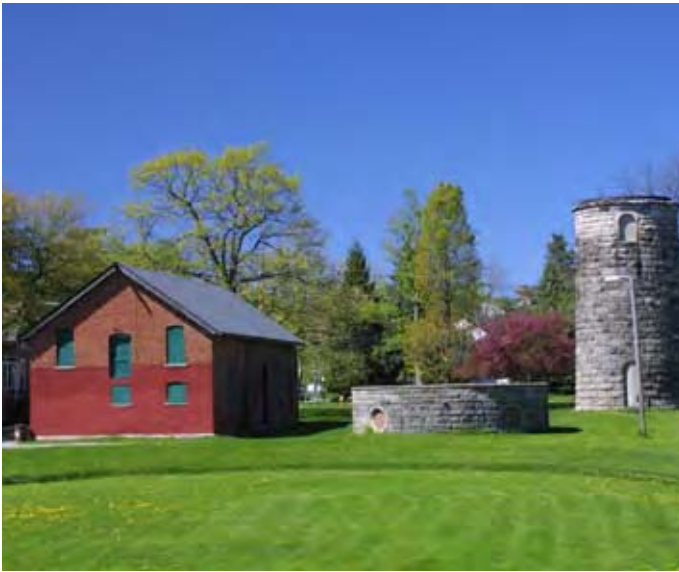
HISTORIC BUILDINGS AT MORGAN STREET RESERVOIR
