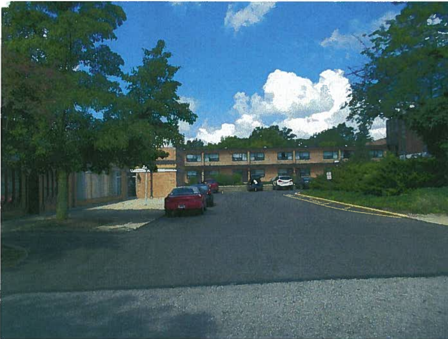
Existing Parking Area Behind Bank and Oberlin Inn
