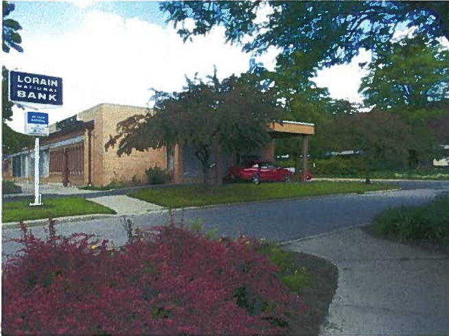
Existing Bank Drive-Through and Access Drive from East College Street
