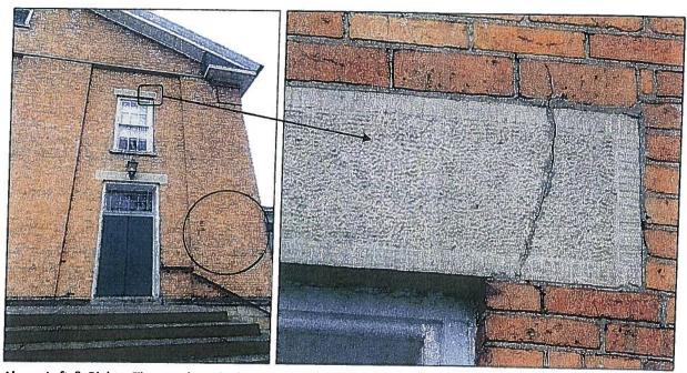
Above Left & Right: The north end of the east elevation has cracking and brick face spalling. The detail of the stone lintel shows that the crack in the stone continues to the brick above.
