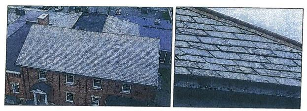
Above Left: The overall view of the slate roof shows no signs of major replacement or repair.
