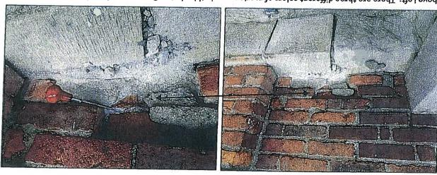
Above Left: There are three different colors of mortar seen in this photo. Gray, tan and an almost white coloring. Above Right: The white mortar seen in this close up is the deepest within the wall structure and is the original mortar. We used an awl to dig into the soft mortar until it supported itself. The outer mortars are repointing and/or repair mortars that are much harder in compressive strength.
