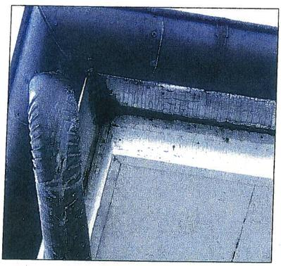
Above: Moisture has wet the backside of this crown molding and softened the wood. Birds, bugs and possibly squirrels have eaten the softened wood, creating a large hole. This area is most likely now a nesting area. Notice that the painted surfaces are very cracked and pieces of brittle paint have fallen off.
