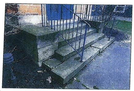
Above: The sandstone steps have deteriorated and the water that has penetrated through to the underlying structure has created damage to the supporting masonry walls. Additional freeze thaw effects have continued to move the stone out of place.
