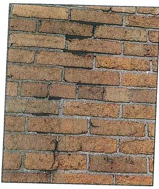
Above: North end of east elevation of Meeting house detail of spalling and cracked brick and mortar.
