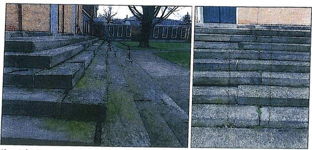
Above Left: The east elevation entrance steps are severely shifted. Most of the original tread stones are reusable.
