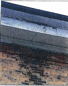
Above Left & Right: The north elevation has areas of staining and wood deterioration in a repeated and uniform fashion. These areas are where the original chimney chases were built into the walls.
