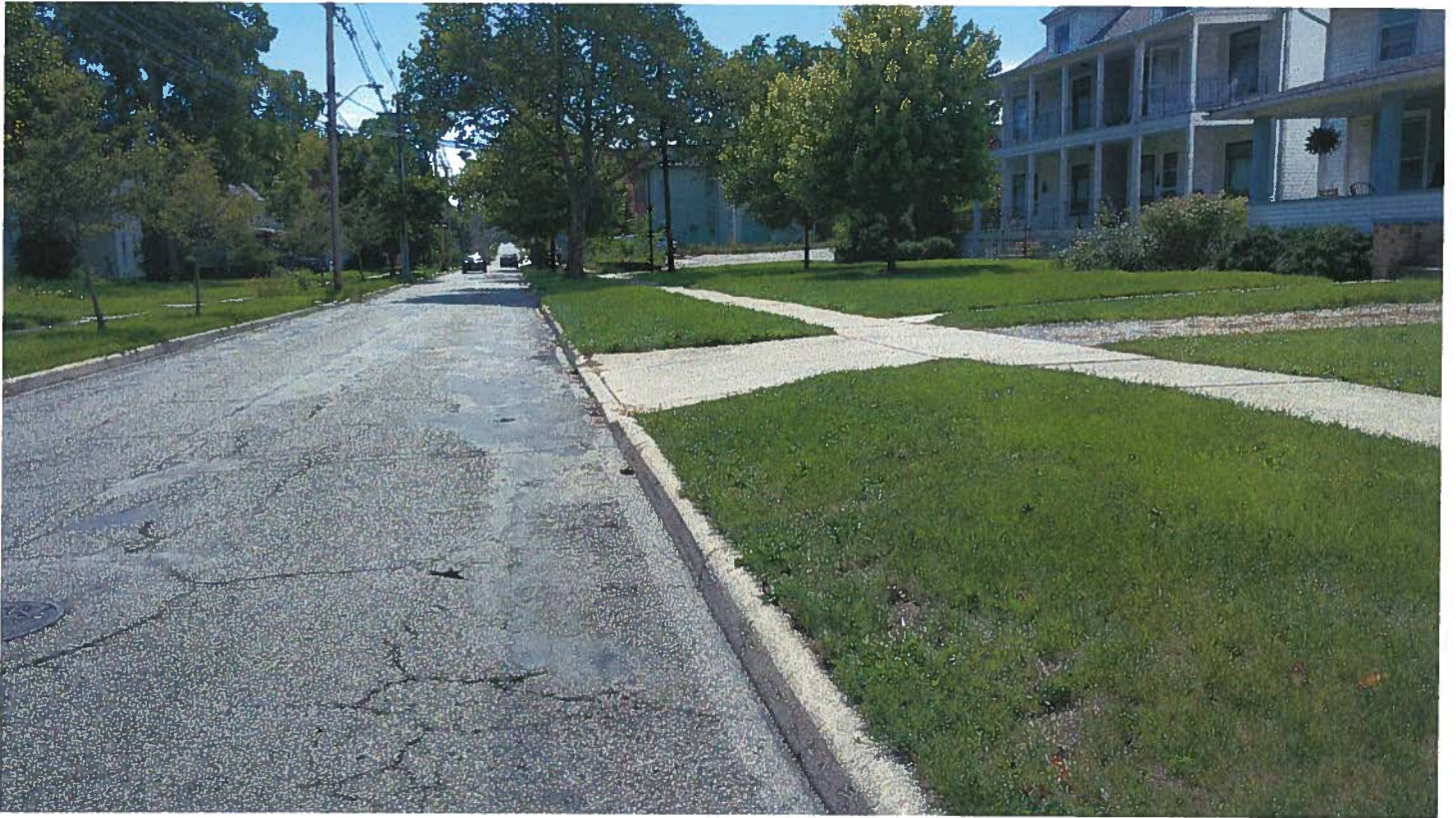
Typical pavement conditions: block, longitudinal and transverse cracking; moderate raveling; small potholes; moderate deformation in wheel travel path; Type 2 curb in good condition.
