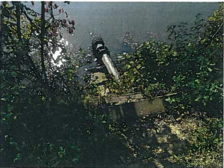
12. The emergency overflow pipe located in Reservoir No. 1.
