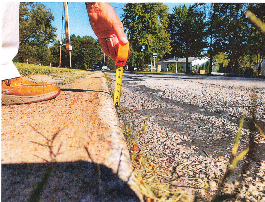
1 3/4" reveal on rolled curb demonstrates the extent to which differential settling has rotated curb away from the roadway. Typical throughout.
