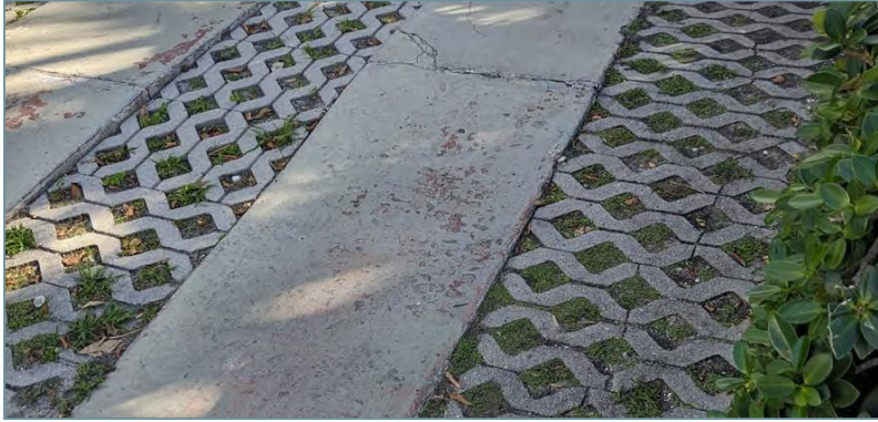
Figure 20: An image of a driveway paver system that may be more stormwater-friendly than traditional paving.
