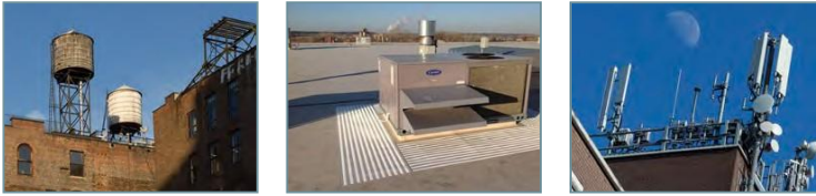
Figure 2: Graphic showing examples of exceptions to maximum height restrictions, including water towers (left), building mechanics (center), and cellphone & radio towers (right).
