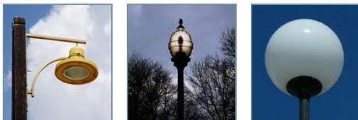
Figure 11: Graphic showing desired downlighting fixtures (left) and undesirable lighting fixtures (right two)
