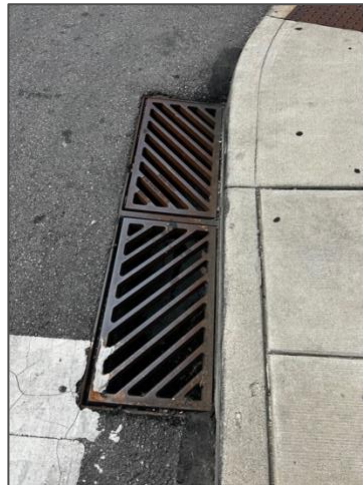
Figure 10: Graphic showing a storm drain incompatible with bike-safe design, as bike tires could fall into slots of storm drain, causing injury.
